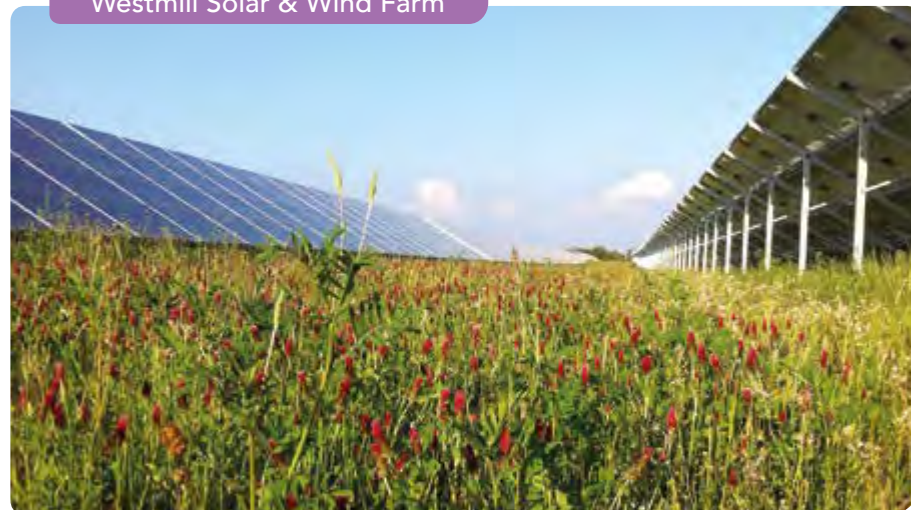
Westmill Solar & Wind Farm
