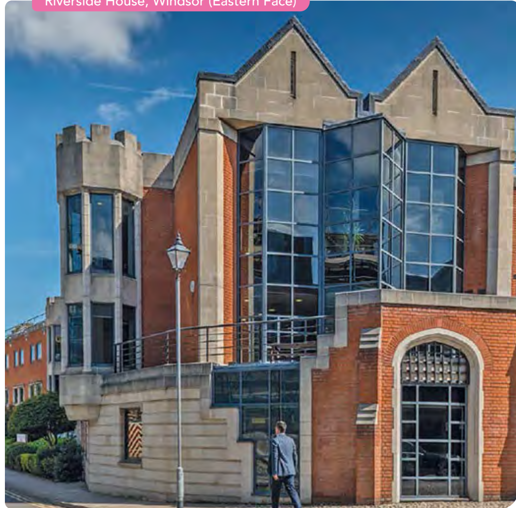
Riverside House, Windsor (Eastern Face)
